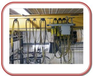
These are the wires that move with the overhead crane.
